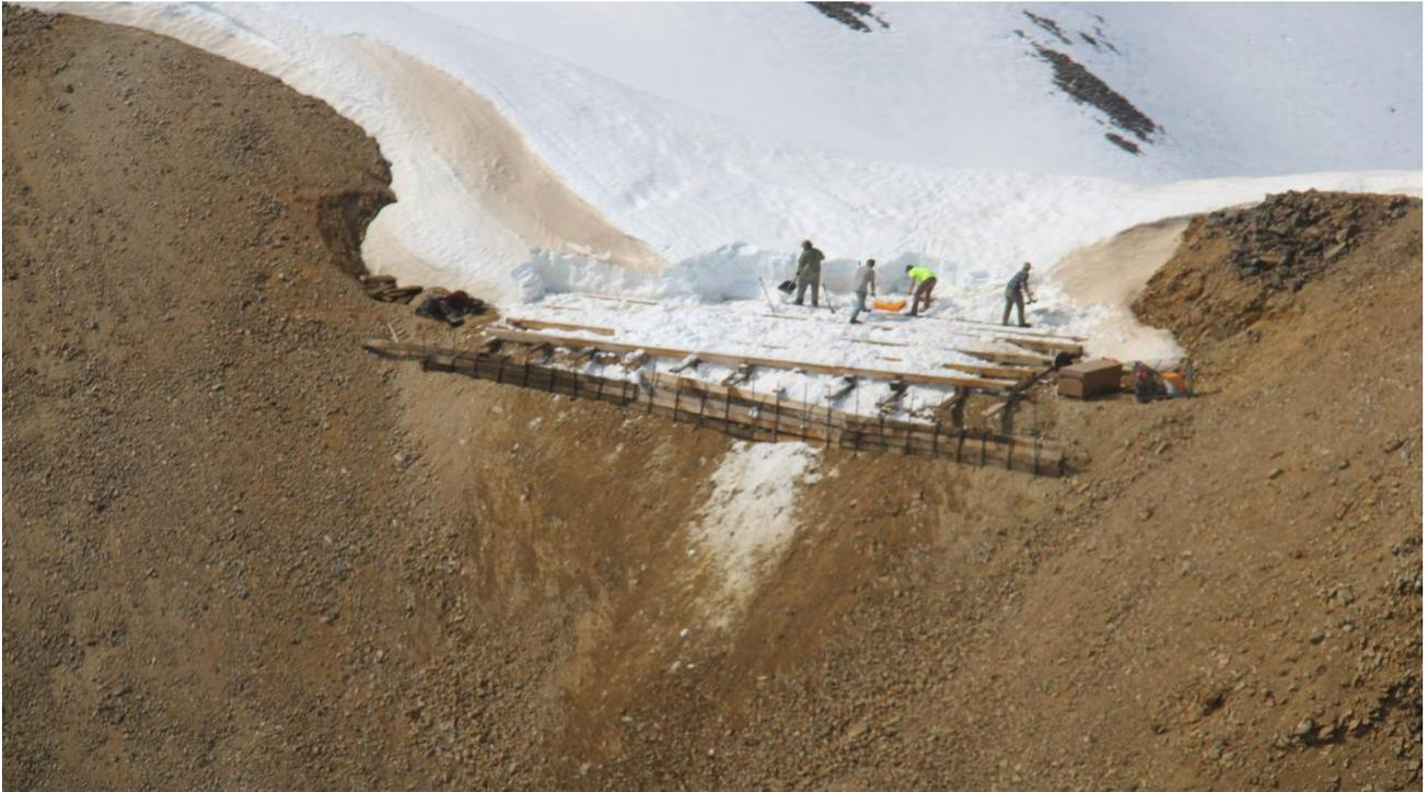
**Figure 3.** Further drill pad being setup at RPM for 3<sup>rd</sup> drill rig later in June 2022
