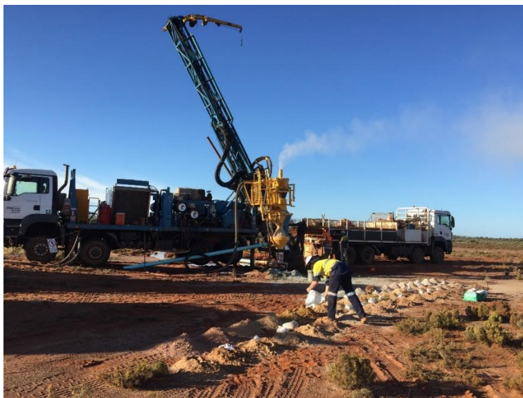
Figure 1 Reverse Circulation Drilling at Apollo Hill
