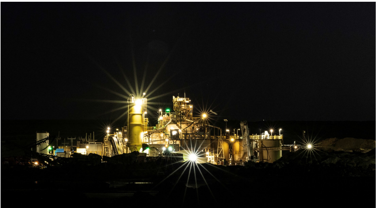
Figure 1: The 1.2Mtpa Lakewood processing facility, Kal East.
