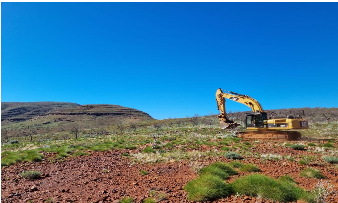
Figure 1 - Earthworks at Hellcat
