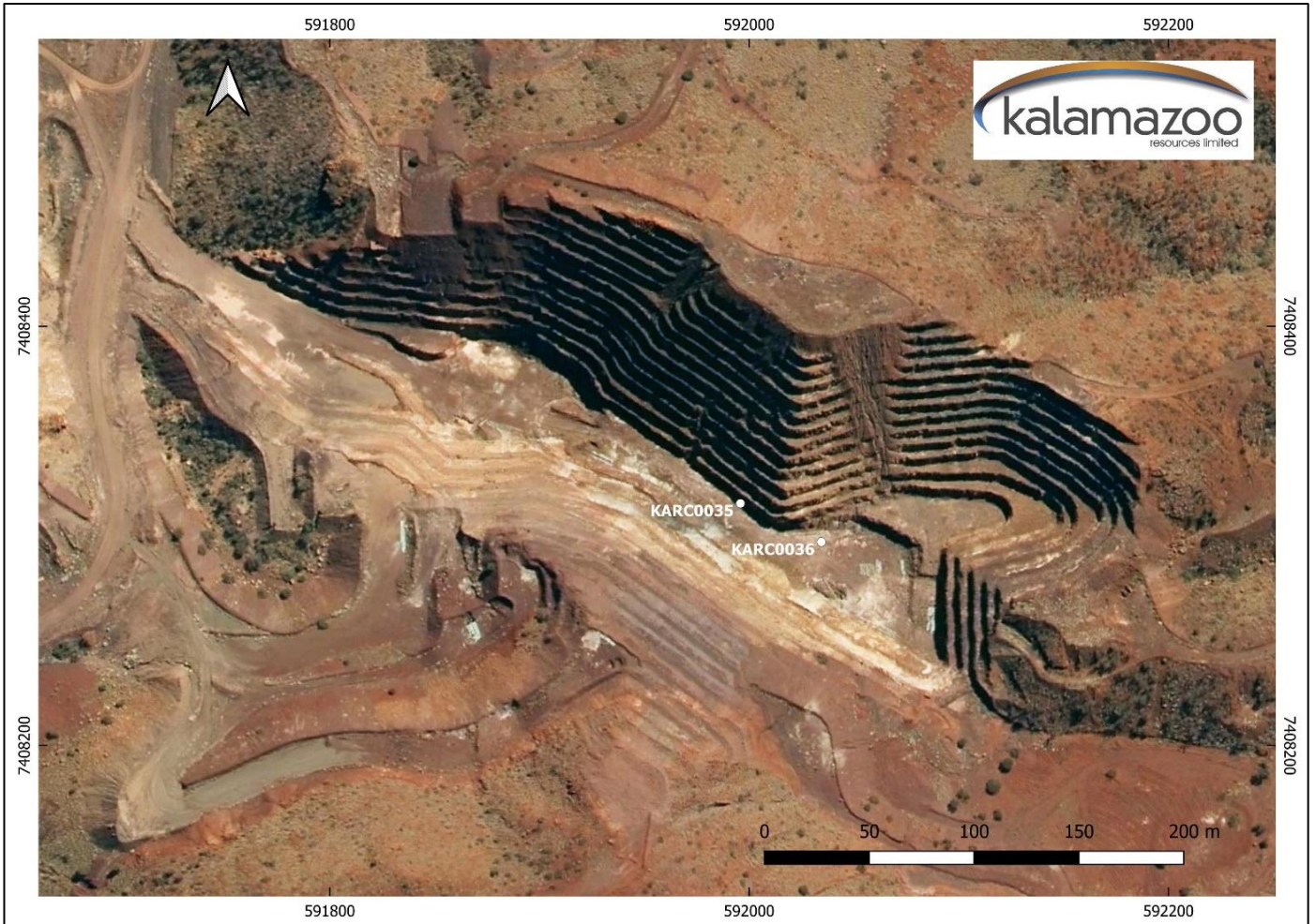
Figure 2: Location plan of metallurgical drill holes within the Mt Olympus open pit
