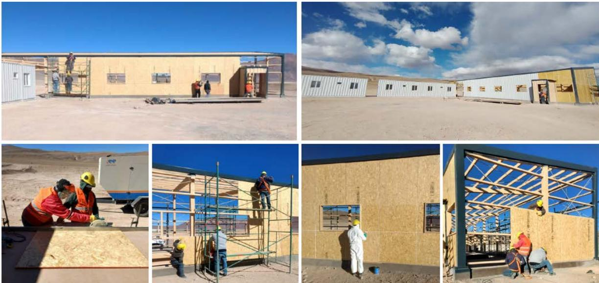
**Figure 2. Rincon Lithium Project – 2,000tpa Operation Site Works in Progress (camp construction works)**
