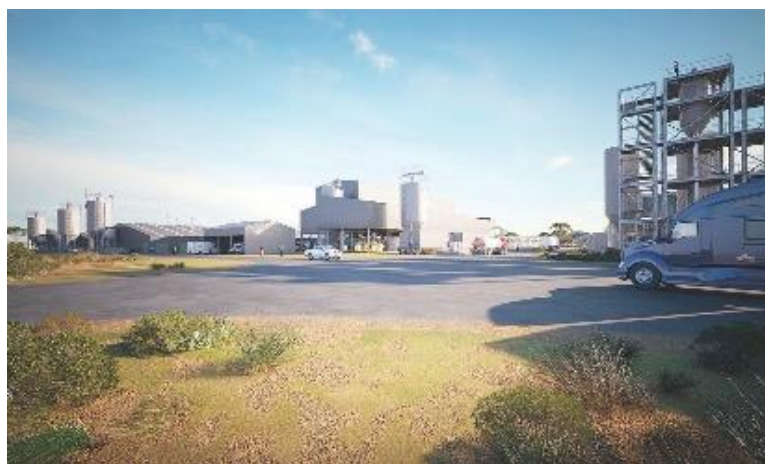
Figure 3. Conceptual illustration of the planned PSG manufacturing facility at Bolivar, South Australia
