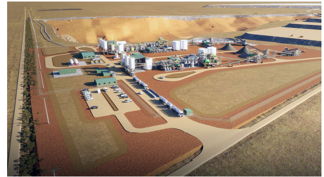
Conceptual illustrations of the maturing engineering design for the upstream operations at Arno Bay
