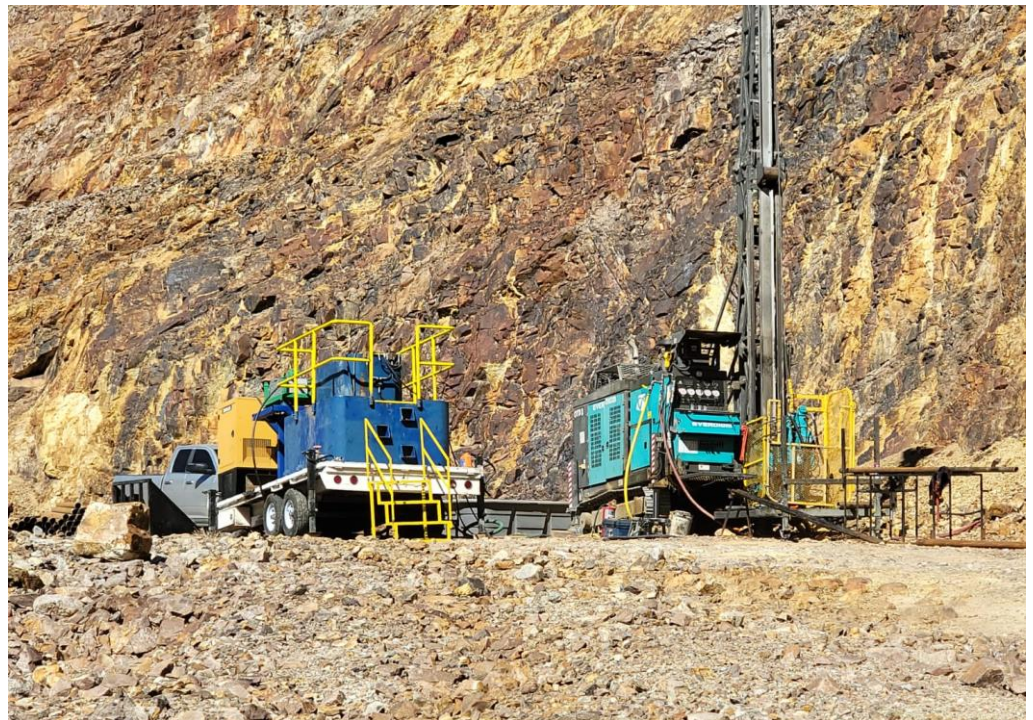
Figure 1: Diamond drill rig on site at Colosseum
